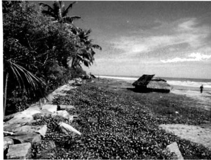
Fig. 54. Of what that is left off the old seawall now located far within the land than the seafront. The beach has grown with sand deposits and presence of beach vegetation is prominent. An unauthorised semi-permanent hut is located on the middle of the beach. (Purakad)
