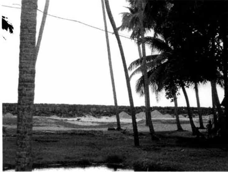
Fig. 29. Piles of sand collected and ready for transportation found adjacent to the seawall at Manakkapadam. The origin of these sand heaps may be the sand within or out of the seawall.
