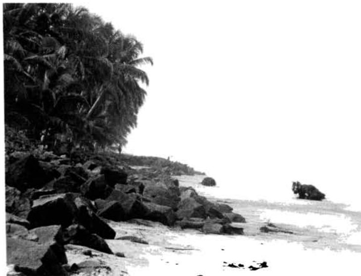
Fig. 31. The view on the southern flank indicates portions of the collapsed seawall and presence of a small flat beach.
