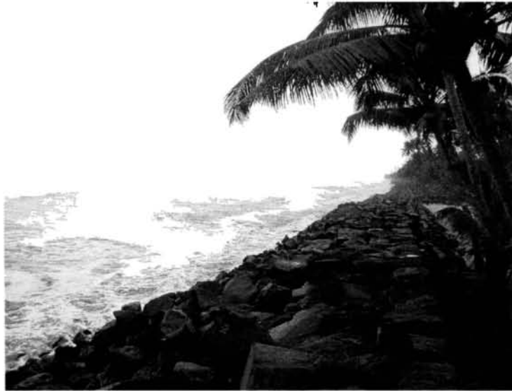
Fig. 24. Further south of Chellanam the Pallithodu seawall protects the northern flank.
