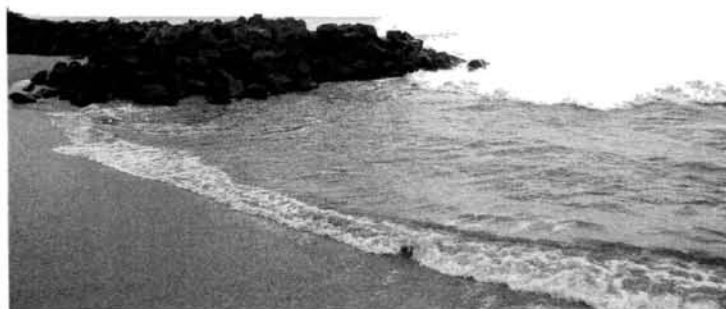
Fig. 25. The sea gap opening at Pallithodu with the collapse of the seawall on the southern tip. This opening permits landing of small fishing crafts with out board engine.
