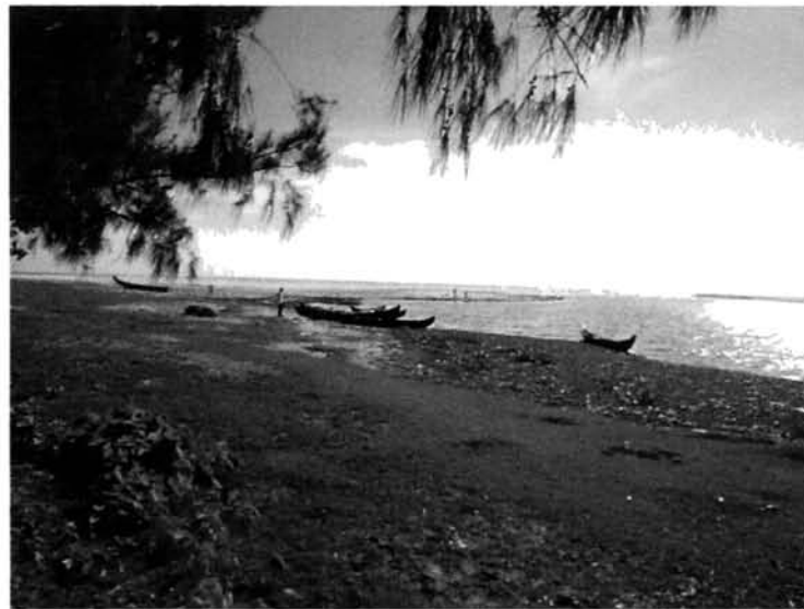
Fig. 57. The closed inlet at Thottappally. Often monsoonal set up piles water above the level of freshwater within the spill way and the operation comes to a standstill.
