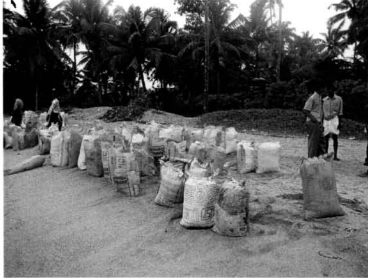
Fig. 26. Artificial beach nourishment by means of sand filled gunny bags as practised at Pallithodu.
