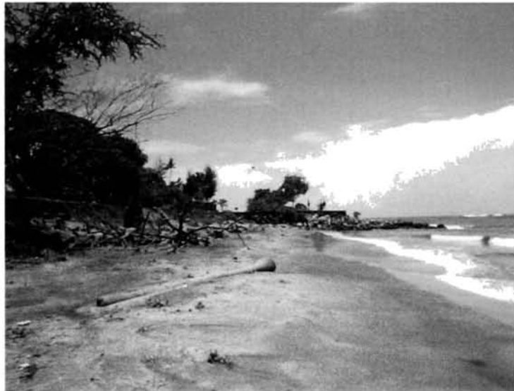
Fig. 15. Same as above where a groyne had restricted the damage.
