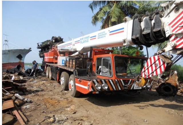
Fig. 3.20 Handling of Main Engine
