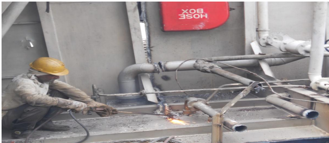
Fig. 3.19 Dismantling of Hull Structure
