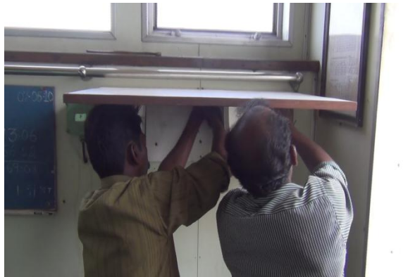
Fig. 3.17 Dismantling of Panelling
