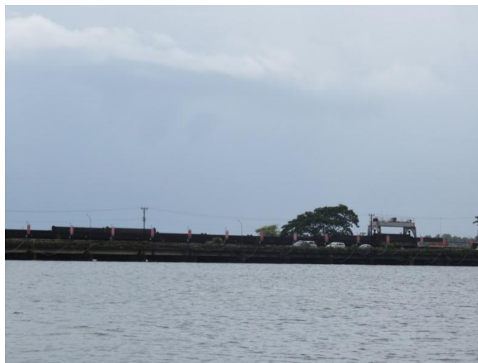
Plate 2.19 Station 6: Thanneermukkom South A view of southern side of Thanneermukkom Barrage
