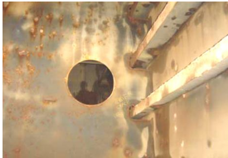
Fig 2.4 (c) Shallow pits < 15% Depth < 1/3 of original thickness
