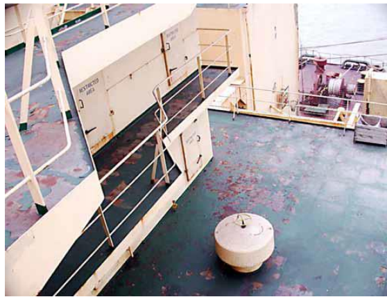
b) Corrosion of super structure
