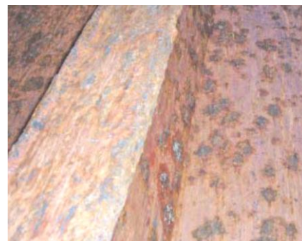
Fig 2.4 (f) Deep pits > 15% Depth > 1/3 of original thickness
