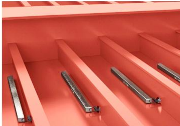
b) Sacrificial anodes in ballast tank of a ship ( http://www.cathwell.com )
