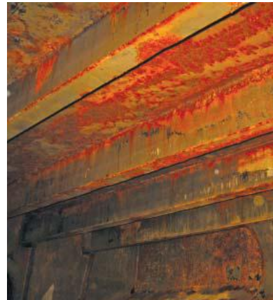
Fig 2.2 (f) General breakdown of coating > 30%
