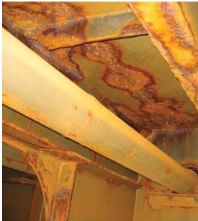
Fig 2.2 (e) General breakdown of coating 20% - 30%
