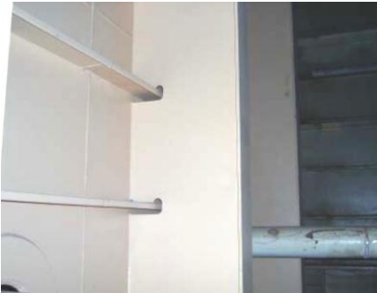
Fig 2.2 (a) Freshly coated, negligible breakdown of coating
