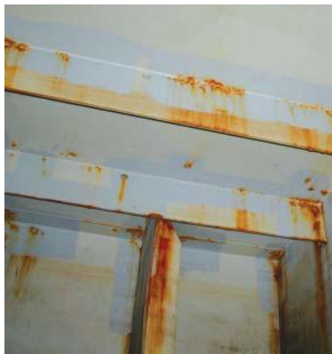
Fig 2.2 (c) General breakdown of coating 5% - 10%
