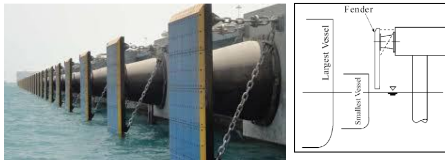
Fig. 1.2 Fenders in a Ship Berthing Structure (courtesy: http://www.portfenders.com )
