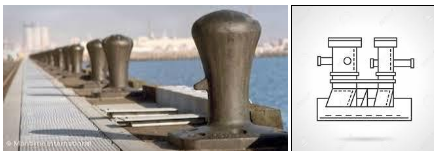
Fig. 1.3 Bollards in a Ship Berthing Structure (courtesy: http://www.popularmechanics.com )
