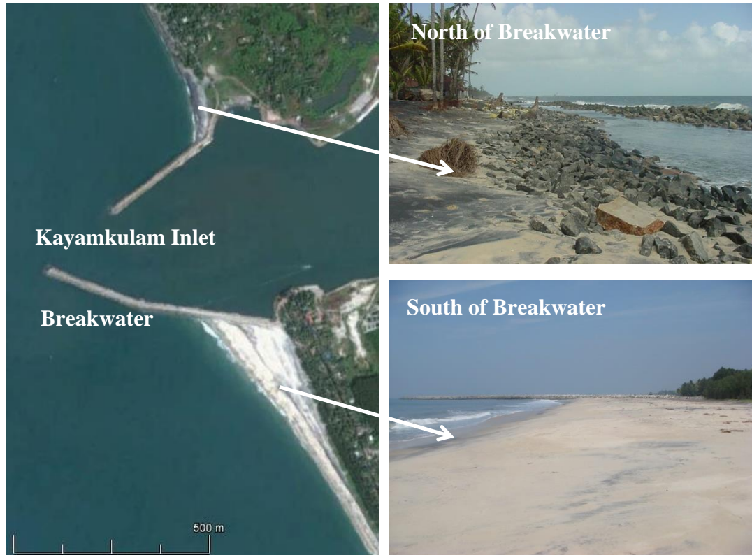
Fig. 5.10 Satellite imagery (Source: Google image) and snapshots showing erosion immediately north of Kayamkulam breakwater and accretion towards south of the breakwater
