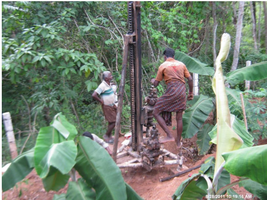
Plate 10 Drilling bore well for water
