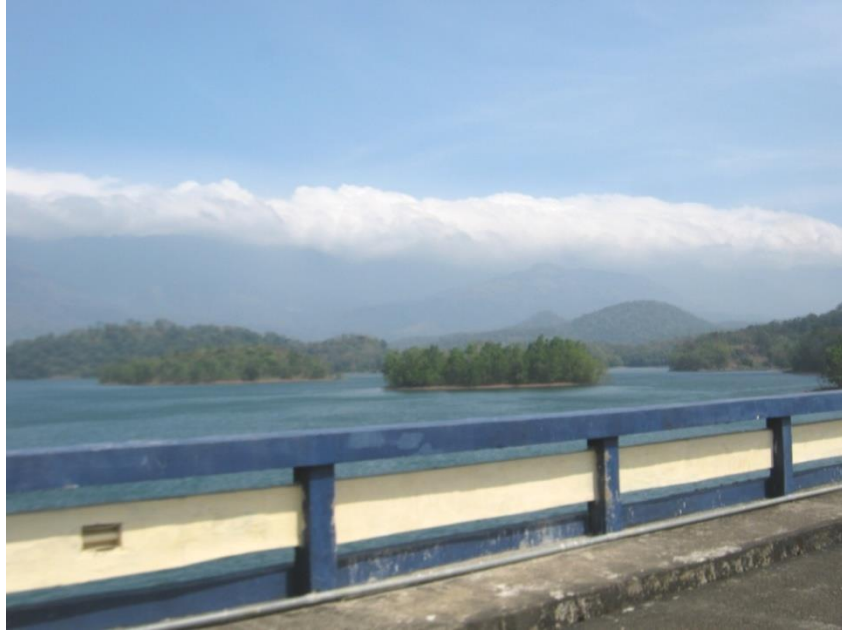
Plate 5 A view of the reservoir of Peppara Dam
