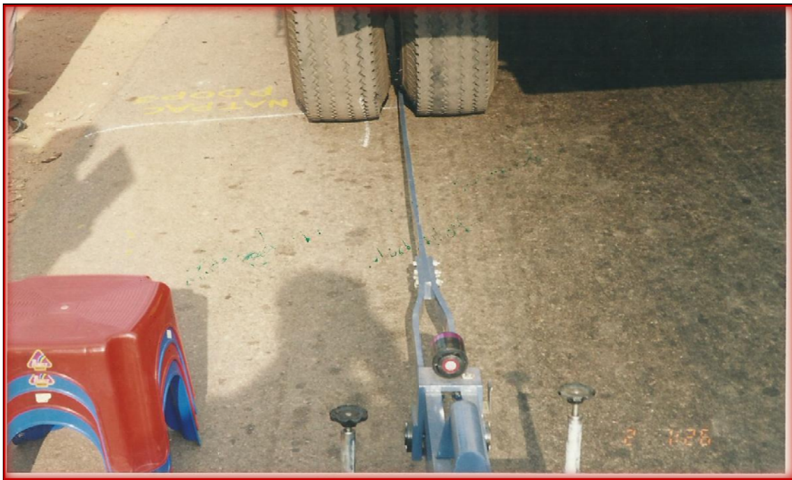
Fig. 3.17: BBD Survey In Progress- Location of Probe
