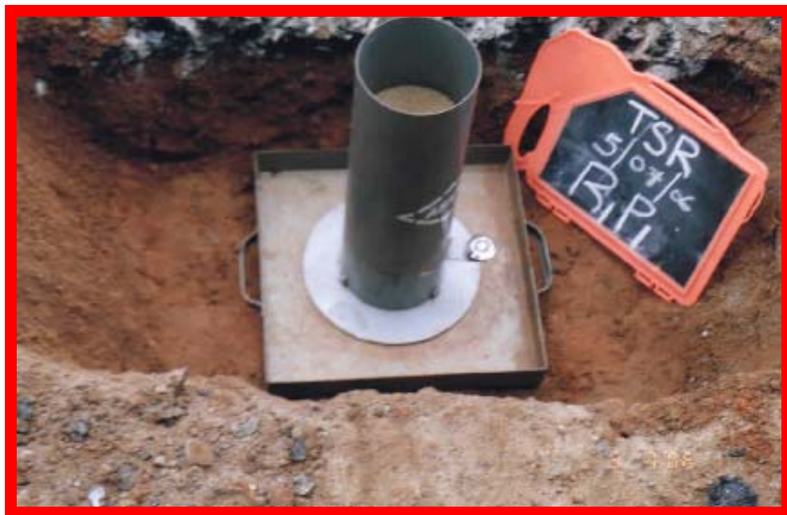
Fig. 3.21: Trial Pit and Sand Replacement Test in progress
