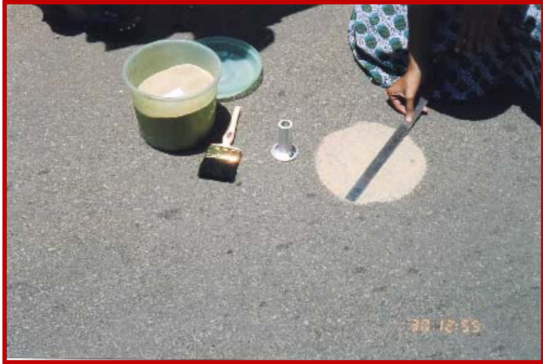
Fig. 3.14 Sand Patch Test in progress
