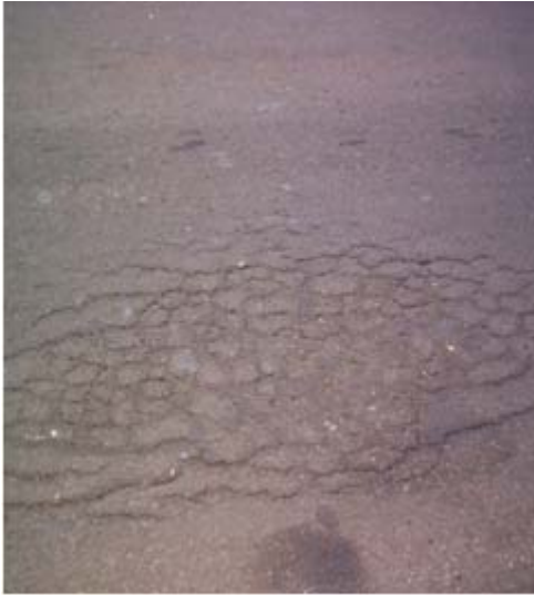
Fig. 3.5 Alligator cracks
