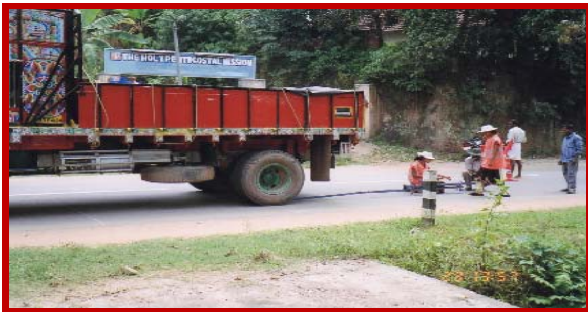
Fig. 3.16 BBD Survey in progress - Deflection Observation point
