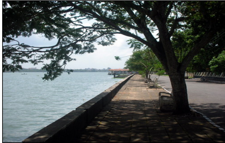
Figure 2.7: Station-5, Cochin Harbour- Embarkation Jetty (CH-EJ)
