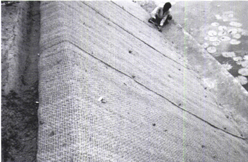
Figure 6.4. Laying of geotextiles on the side bank of the pond
