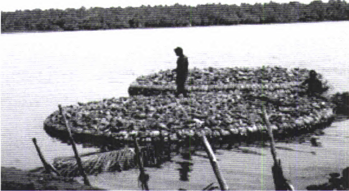
Figure 5.2 Retting of coconut husk
