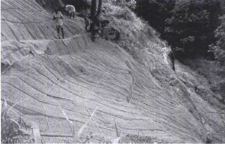
Figure 5.5 Laying of coir geotextiles on rock surface
