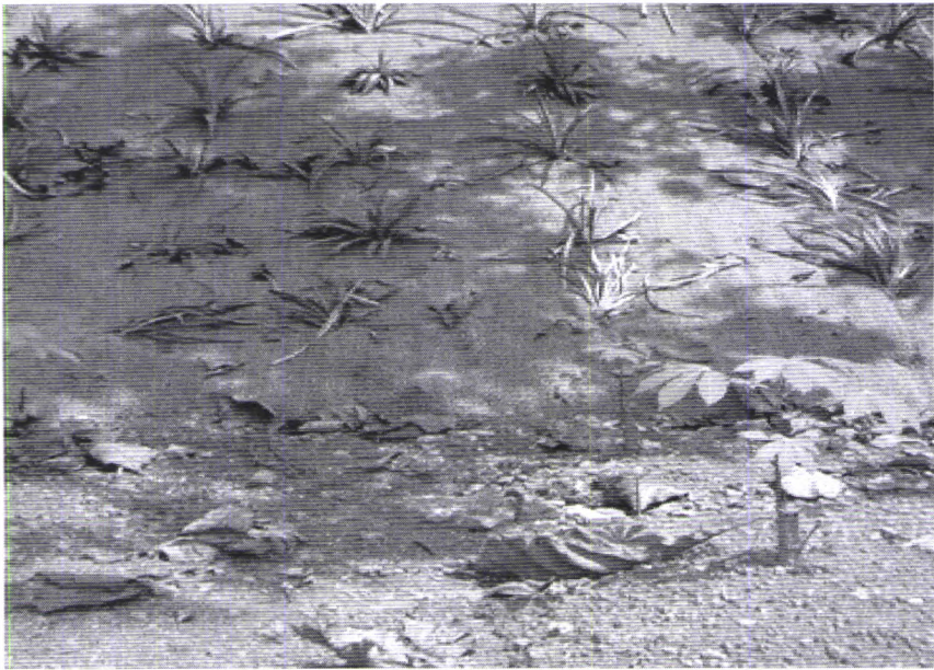
Figure 6.20. Slope treated with coir geotextile planted with pineapple and tapioca on the terraces
