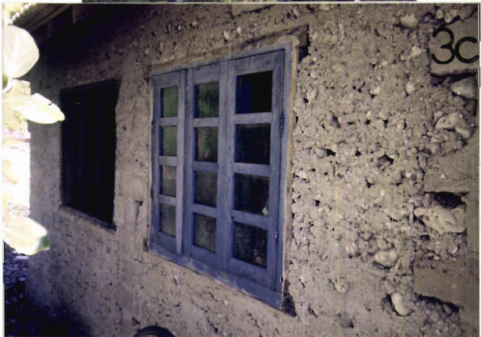
Photograph 3b & c.: Buildings constructed with coral stones.
