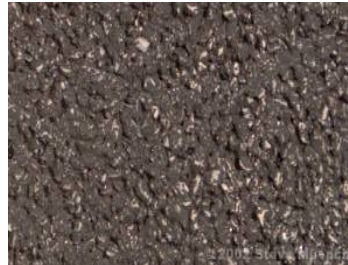
Fig. 2.3 Open graded HMA
