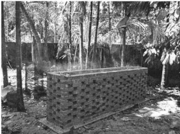
Figure 6.11 Brick kiln enclosure for burning rice husk
