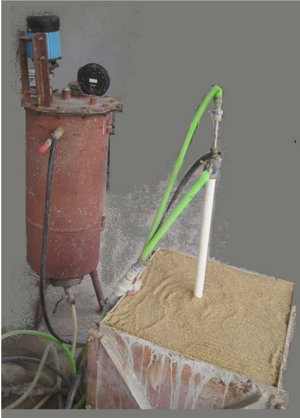
Fig. 5.4 Grouting set up
