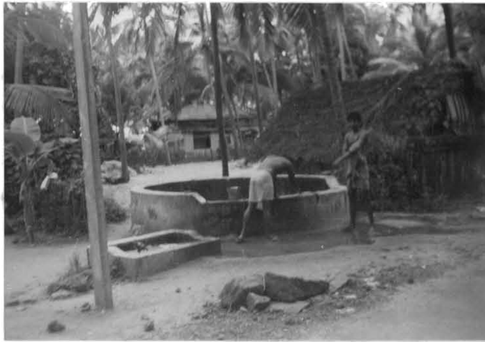
PHOTOGRAPH - 5 TYPICAL COASTAL WELL
