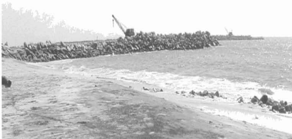
Fig. 1.6 Impact of breakwater on longshore transport of sediments at Kayamkulam inlet. Accreted beach observed in the south of breakwater (a) and eroded beach formed in the north (b)
