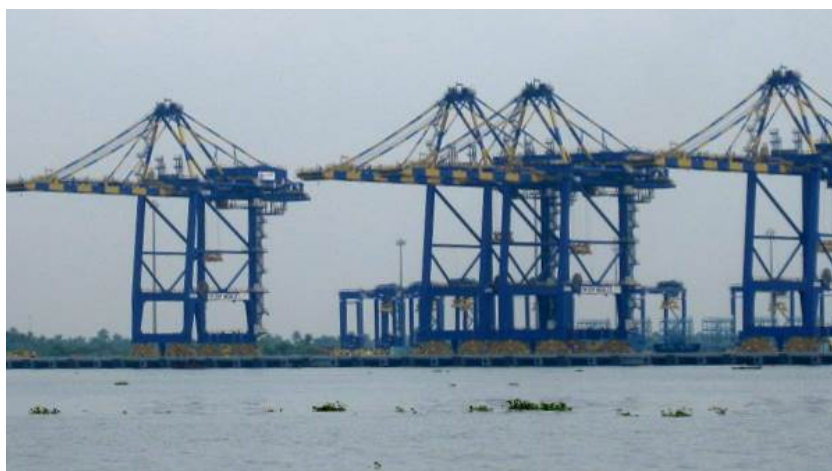
Plate 2.11 Station 5- Vallarpadam-Bolgatty Construction phase of Vallarpadam ICTT during the sampling period.
