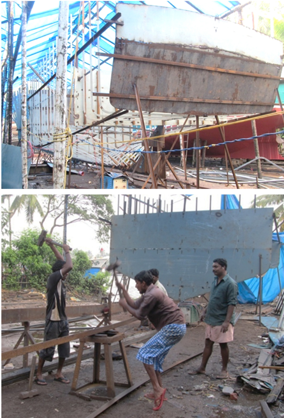
Fig. 4.2 Construction of a steel trawler
