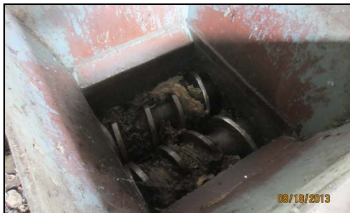
Figure1.2 Scrolls of the pre-breaker
