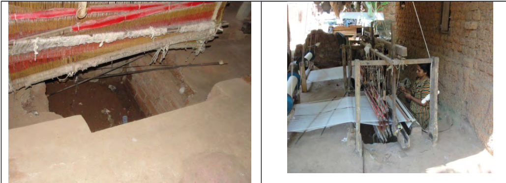
Inside view of Ooruttabalam Society in TVM. The pit is wet, especially during rainy season.
