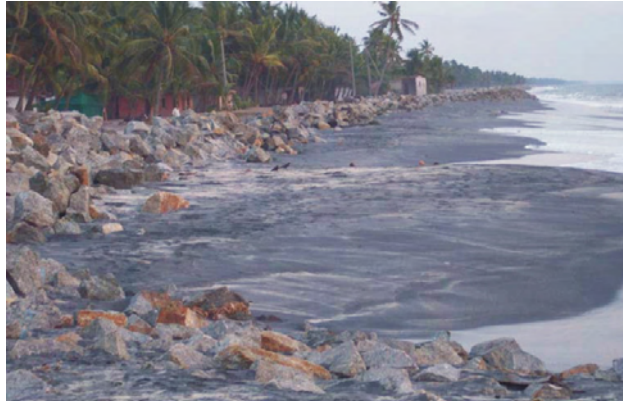
Figure 1.7: The islets of Alappad and Arattupuzha are made up of rich black sand deposits. It is evident that the sea wall is not a viable defense against the sea.
