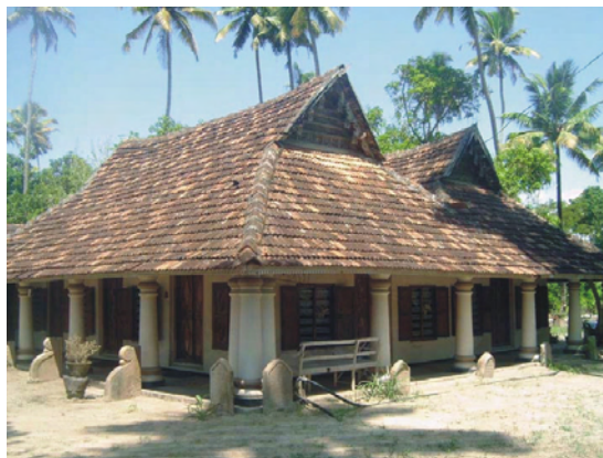
Figure 1.15: The coastal belt is steadily sinking across time- This house has evenly subsided to a depth of 20 cm during its 200 years of existence (Achari, 2005).
