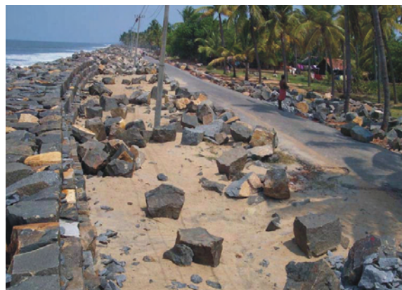
Figure 1.6: The huge boulders of the sea wall were flung away by the tsunami
