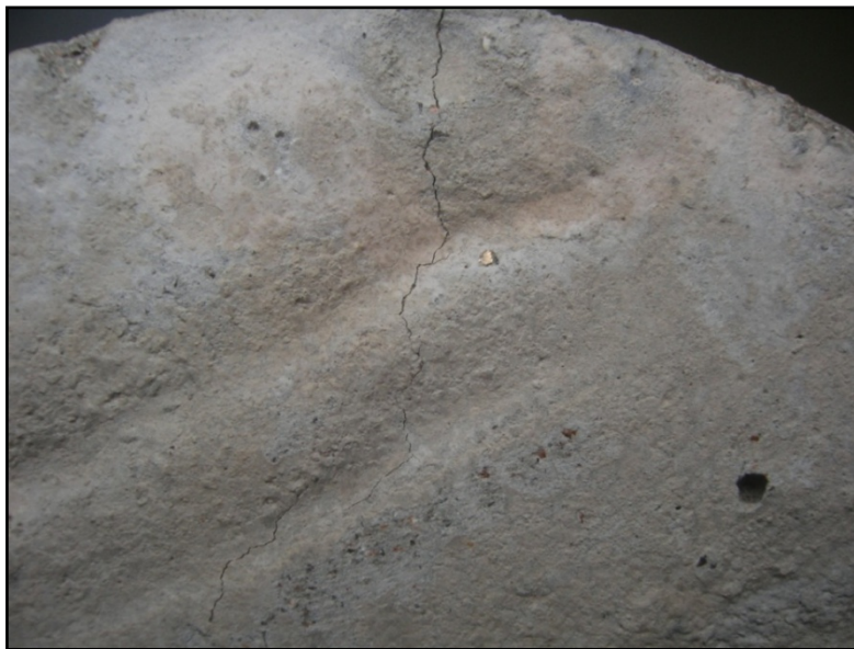
Figure 6.71 Typical major crack in CC heated to 600°C-overall view.
