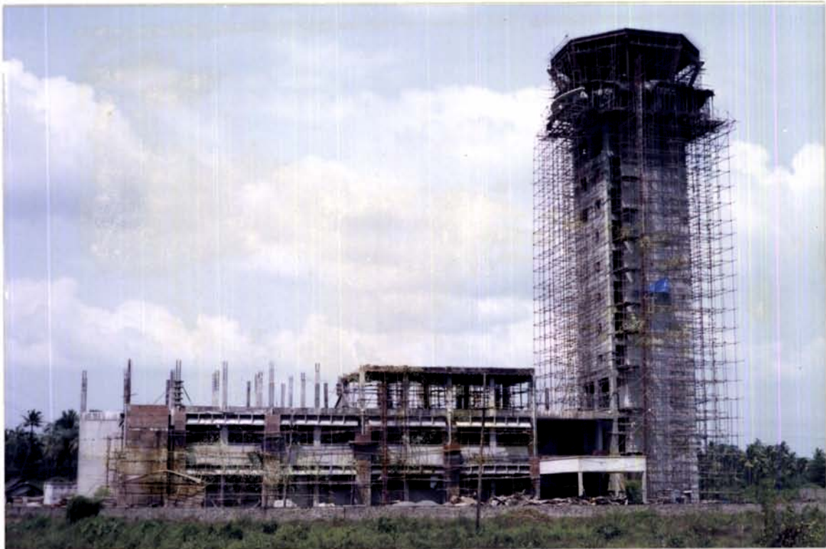
AIR TRAFFIC CONTROL TOWER - UNDER CONSTRUCTION
