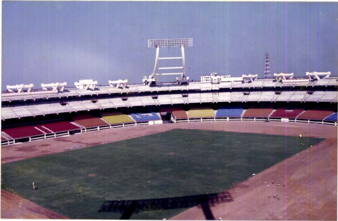
INSIDE VIEW OF THE JAWAHARLAL NEHRU INTERNATIONAL STADIUM AT COCHIN
