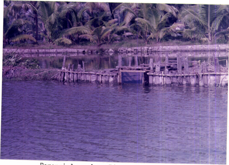
Perennial pond at Edavanakkad with the sluice opening to the feeder canal.
