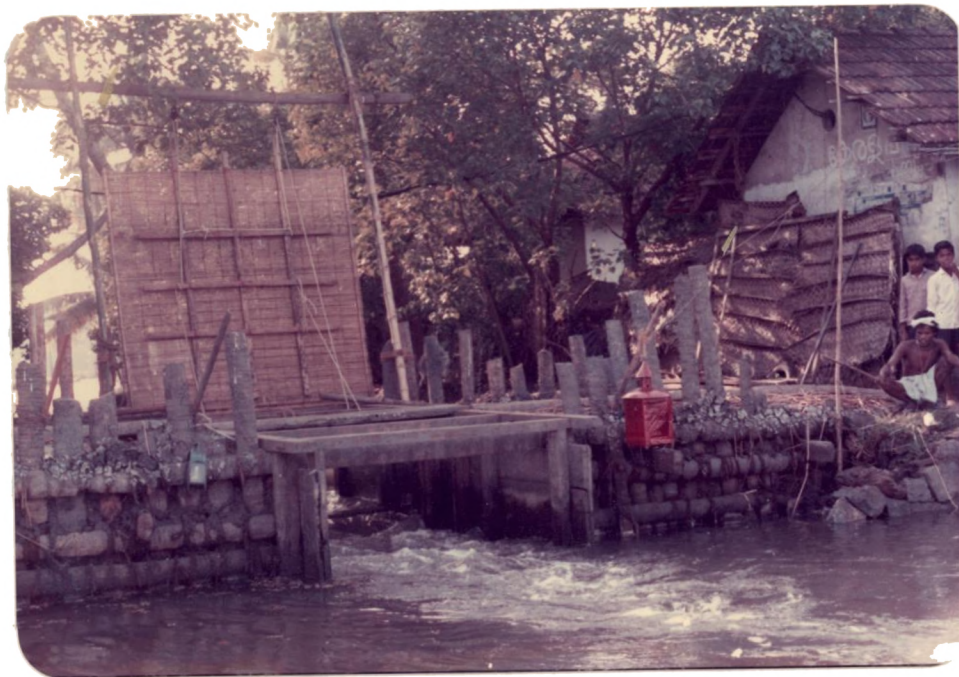
B - Wooden sluice gate with accessories
