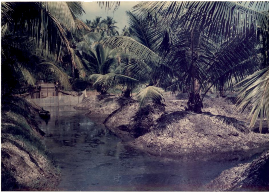
B - Sluice gate with nylon screens and filters
