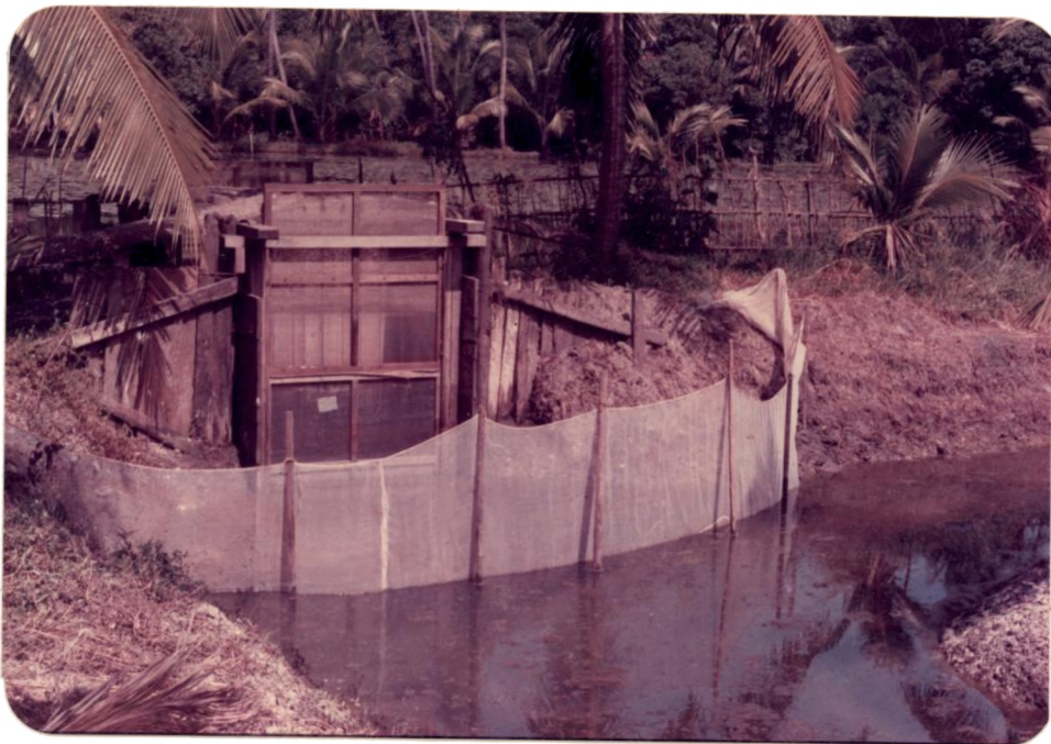
B - Nylon mesh screen in front of sluice gate to prevent predators
