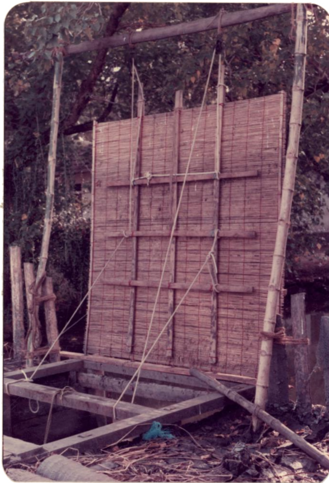
B-Wooden sluice installed and adichil suspended for drying
