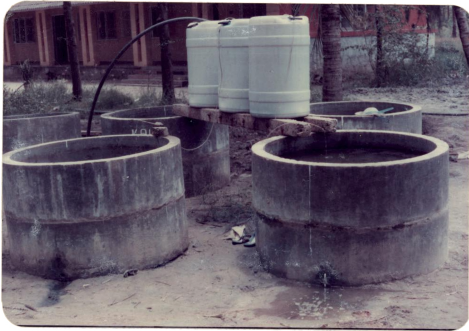
A - Conditioned circular cement tanks
