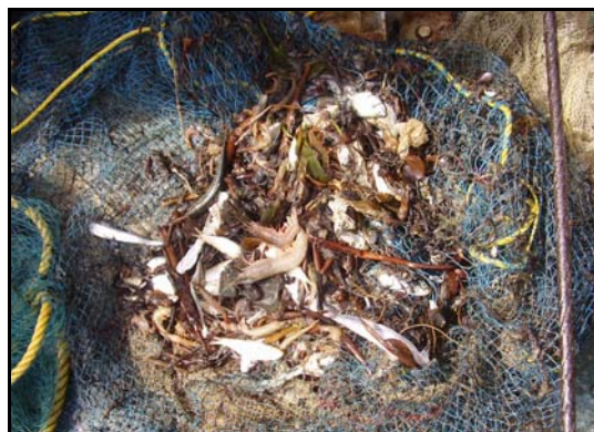
Fig 8.1 Blockage in the Separator panel-40 S
